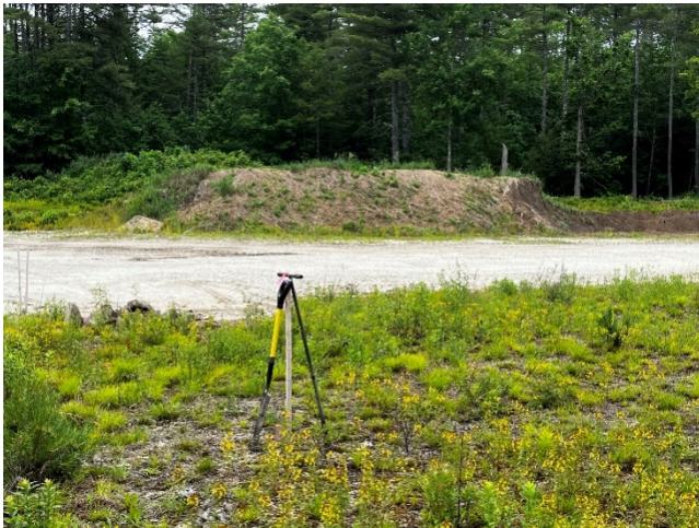
Views of topsoil stockpile along the northern boundary of the excavation
